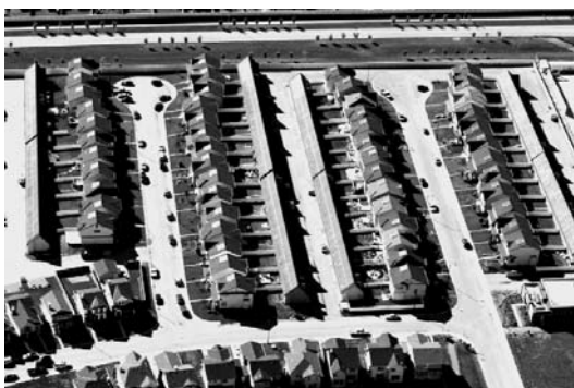
Figure 7.13: Okotoks complex (Canada)
