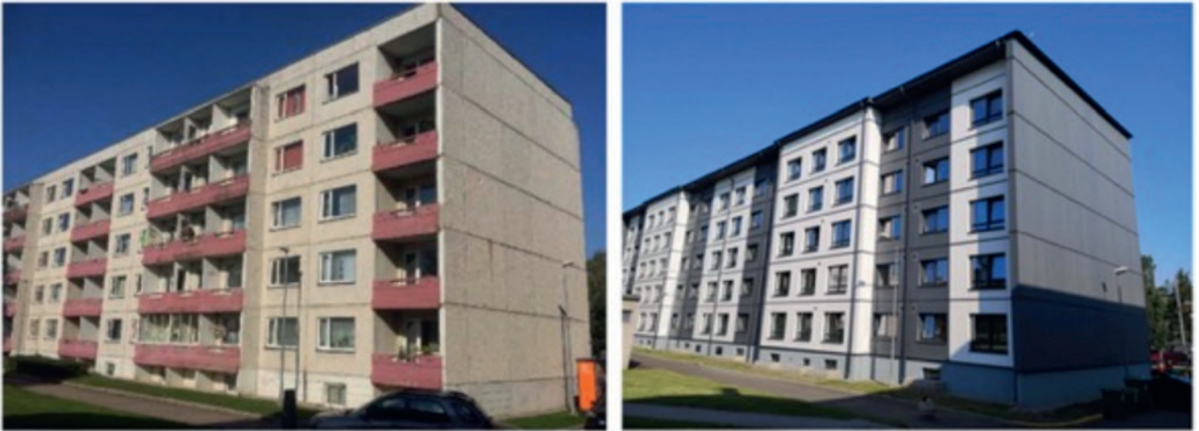
Figure 5 Apartment building in Estonia before refurbishment in 2015 (left) and after a low-energy refurbishment in 2018 (right) (source: Hamburg et al. 2020 ).
