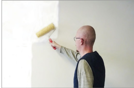
Figure 17 | Repainting with light colour can significantly improve the lighting conditions in rooms. [© Fraunhofer IBP]
