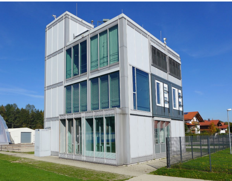
VERU Modular Test Facility for Energy and Indoor Environment Investigations — façade view © Fraunhofer IBP
